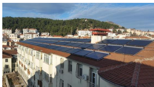
Image 1: Solar collectors in Mamatseio Hospital
